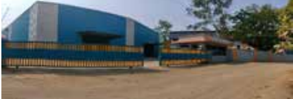
Khopoli, Maharashtra Installed capacity of 80,000 MTPA
